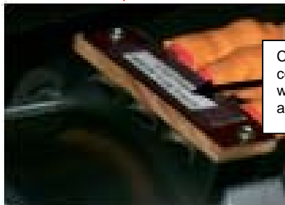
Phase Cable Connection at Alternator
